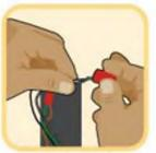
insert the wires into wire nuts.
