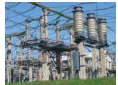
Figure 2 Transformers at this substation step down the voltage so that it is low enough to be transmitted to neighbourhoods.
