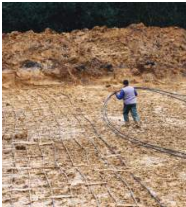
Figure 1 Pipes are buried underground to allow for the exchange of thermal energy between an antifreeze–water mixture and Earth.
