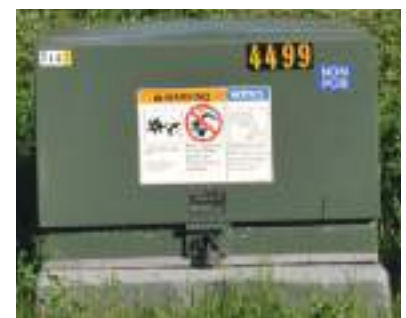
Figure 3 This residential transformer steps down the voltage to 240 V for use in your home.
